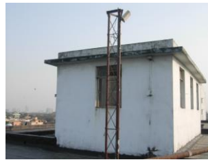
Fig.5 Antenna MAST at Palit Building Rooftop
