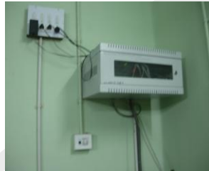
Fig.8. Switch mounted in a box for 5.8 GHz to LAN converter
